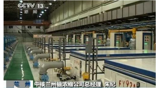
China's Lanzhou Enrichment Plant
