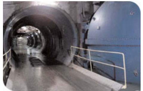
One of the bulkhead doors at Cigar Lake could not be sealed. As a result, the underground development is being allowed to flood. Courtesy: Cameco Corp.
